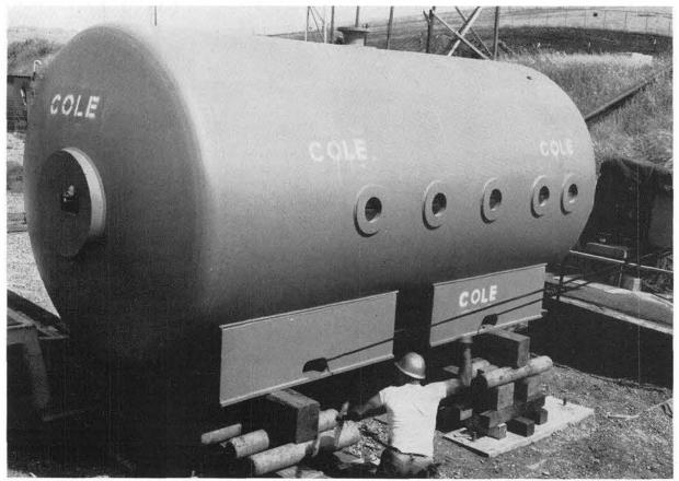
FIRING CHAMBER for explosive studies at Livermore Laboratory is unloaded at Area 8. The 80,000 pound tank went into operation this month for
